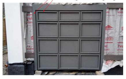
Facade, aluminium frame and aluminium grid is on one plane.
